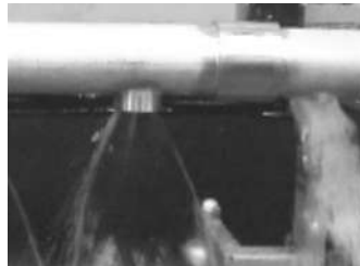
Foreign objects inside the pipe are flushed out through the drain.
