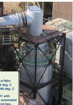
(5) Gas volume: 120,000 m<sup>3</sup>N/hr Inlet temperature: 400 deg. C Outlet temperature: 200 deg. C
