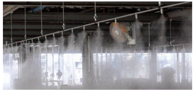
▲Using explosion-proof fans to spread more mist towards operators
